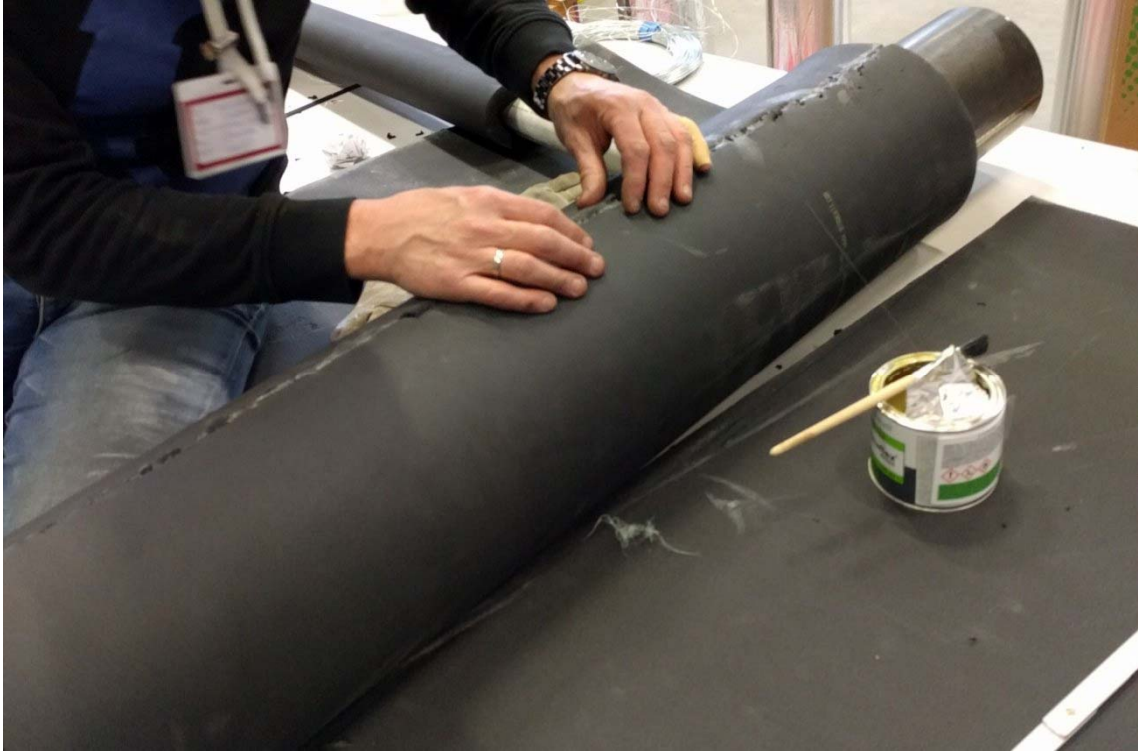
Photograph 1 Installation of the Armaflex
