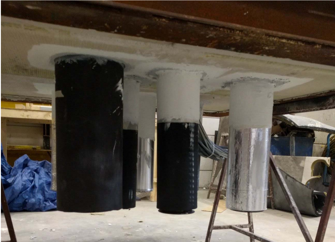
Photograph 3 Overview of the exposed side after mounting the services
